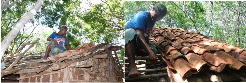
Figura39: Formas de colocar as telhas
